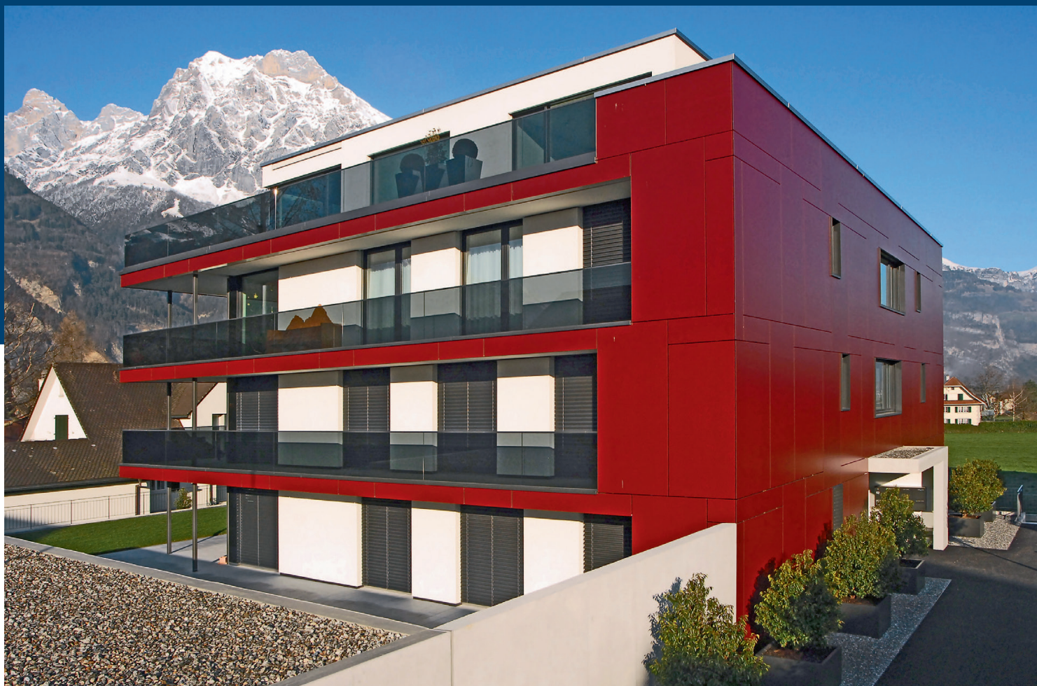
Bahnhofstrasse 52, MFH Brand, Altdorf. Foto: Foto&Grafic Joe Müller, Altdorf Bahnhofstrasse 52, Immeuble collectif Brand, Altdorf. Photo: Foto&Grafic Joe Müller, Altdorf Bahnhofstrasse 52, Casa multifamiliare Brand, Altdorf. Foto: Foto&Grafic Joe Müller, Altdorf
